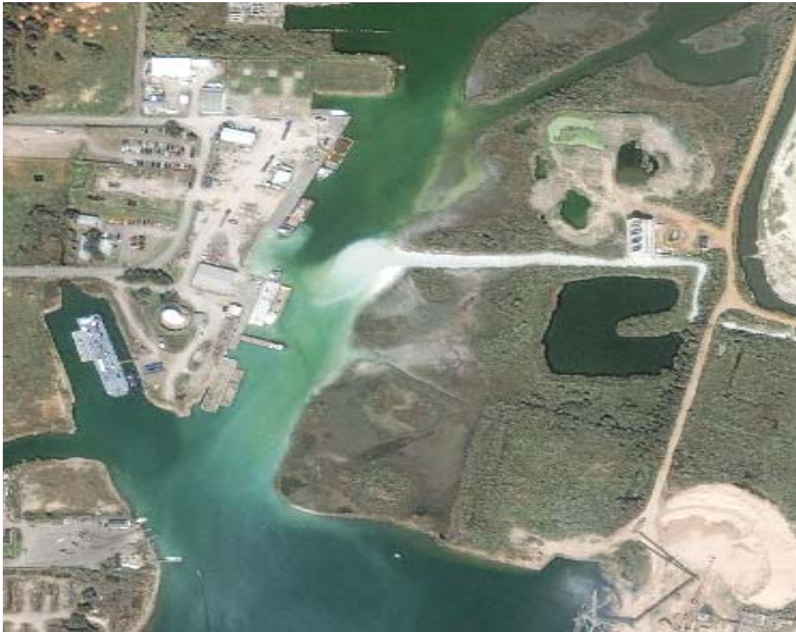
Photo 4: Discharge emanating from MPC's Outfall 003 due to emergency upset conditions, (October 2002)
